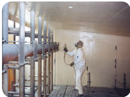
FIGURE 2 Conventional spray application of epoxy vinyl ester polymer lining.
